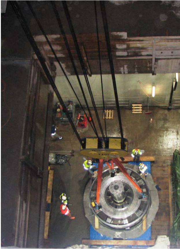
Figure 10 & Figure 11: Lowering of the Last Deflector
